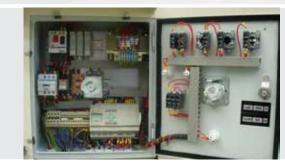
Electric panel with overload protection elements and integrated controls
